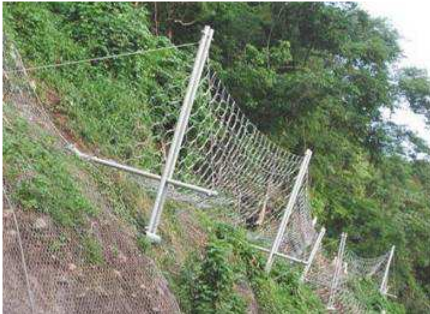
Installed Rock Barrier Fence and Rock Curtain
