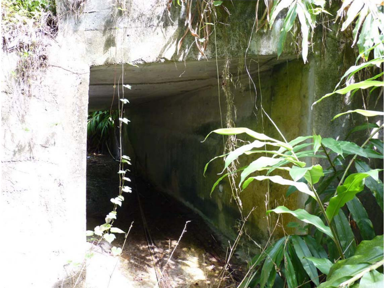
Figure 22 : Photo of Box culvert
