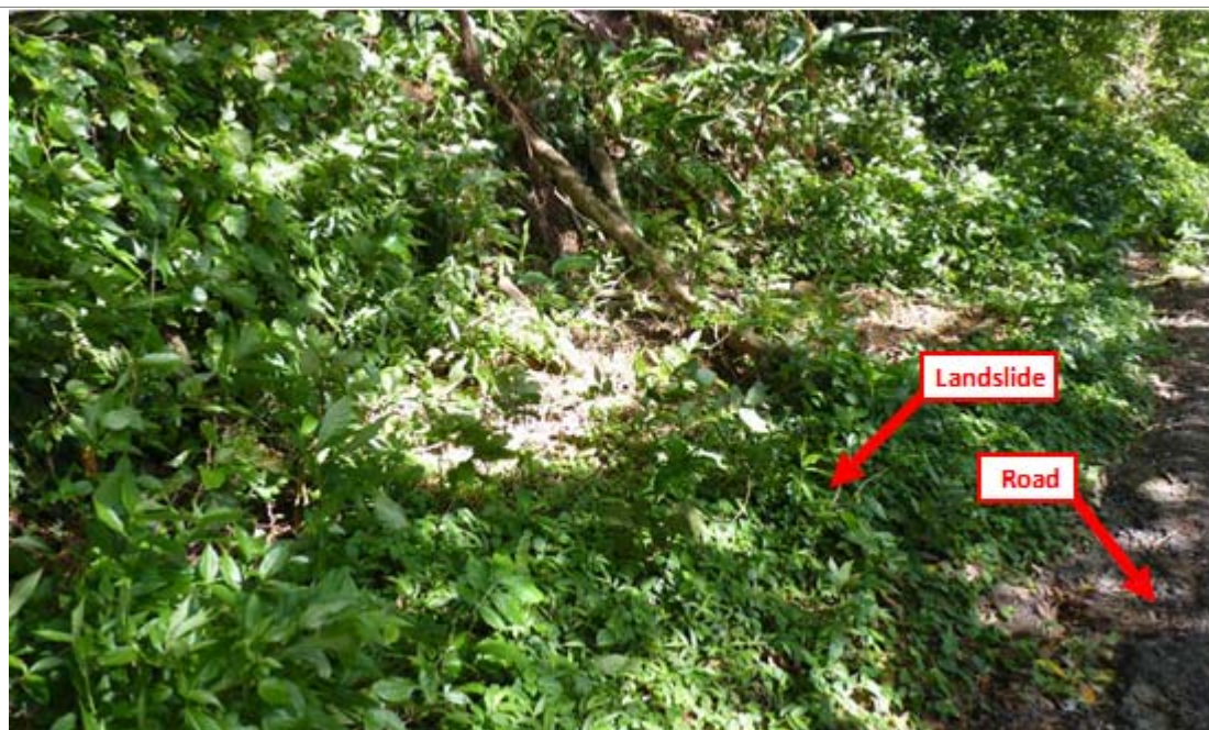
Figure 36 : Landslide on a cutting in the side of the road, covering the roadside drainage
