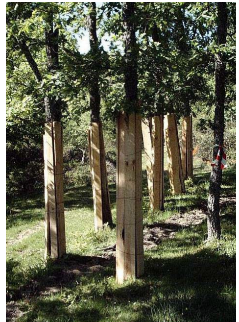
Figure 56: Example of tree protection
