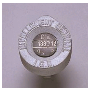
Figure 9: Picture sample of benchmark type "medaillon"
