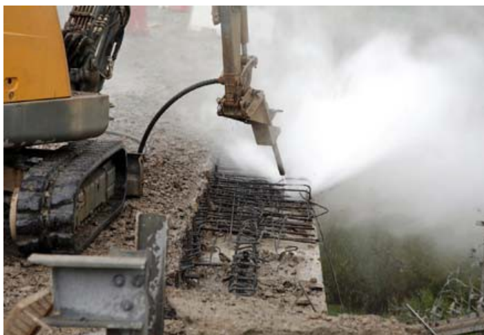
Figure 50 : Left: Demolition of a bridge slab. Right: Debris truckload
