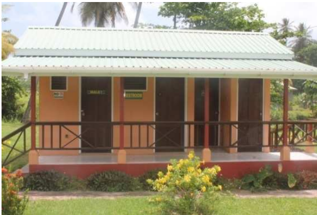
Existing wash room facility
