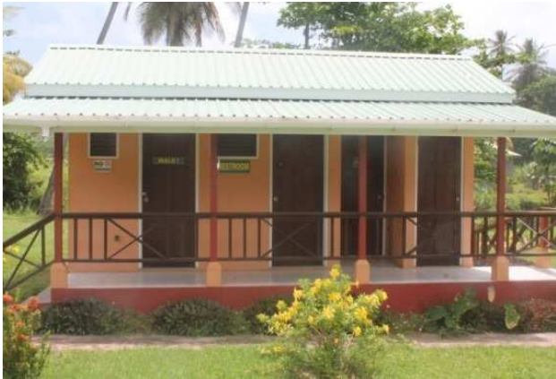
Existing wash room facility
