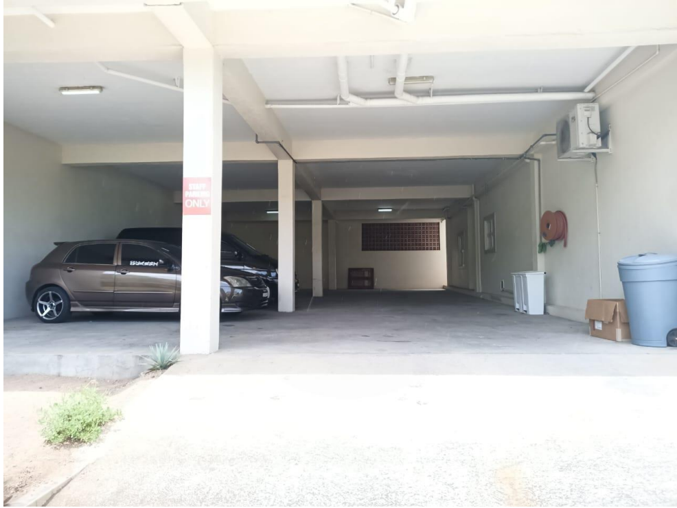
Figure 4. Carport area to be renovated
