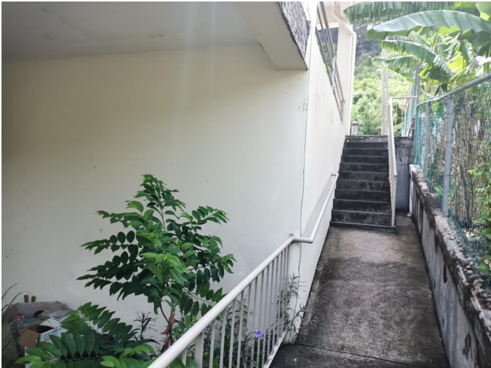
Figure 7. Existing railing to be removed
