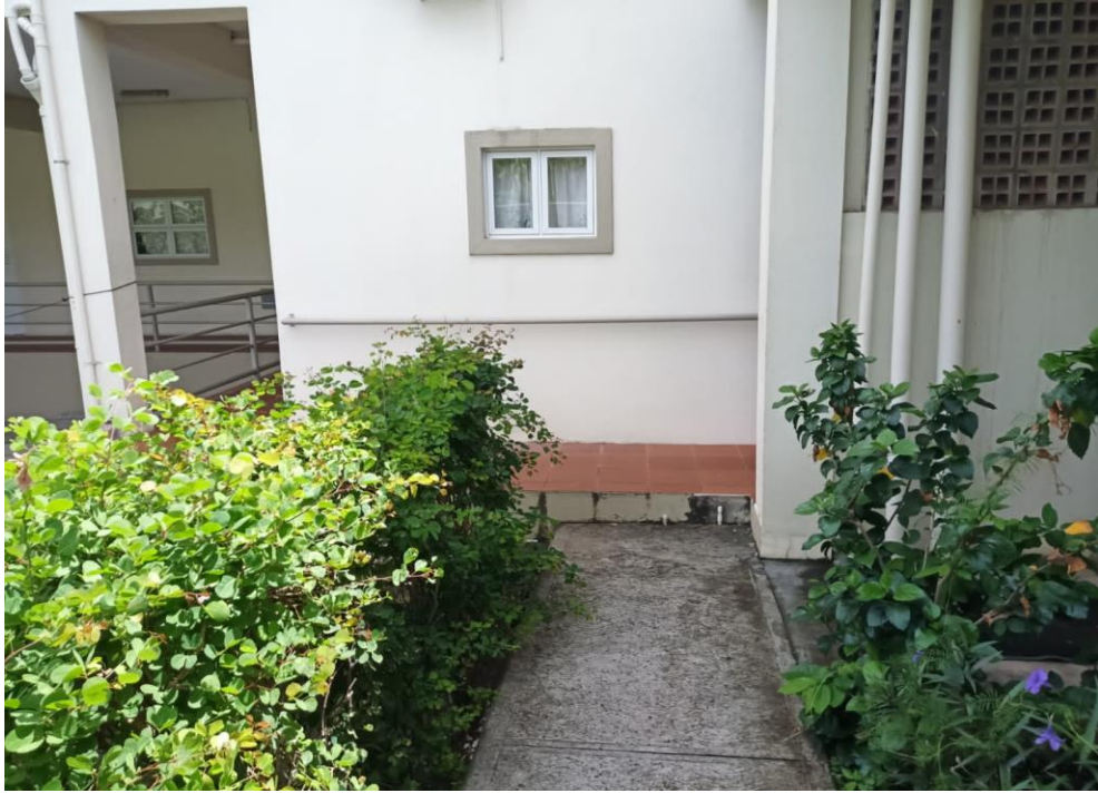
Figure 6. Portion of elevated walkway tiled in brown to be removed
