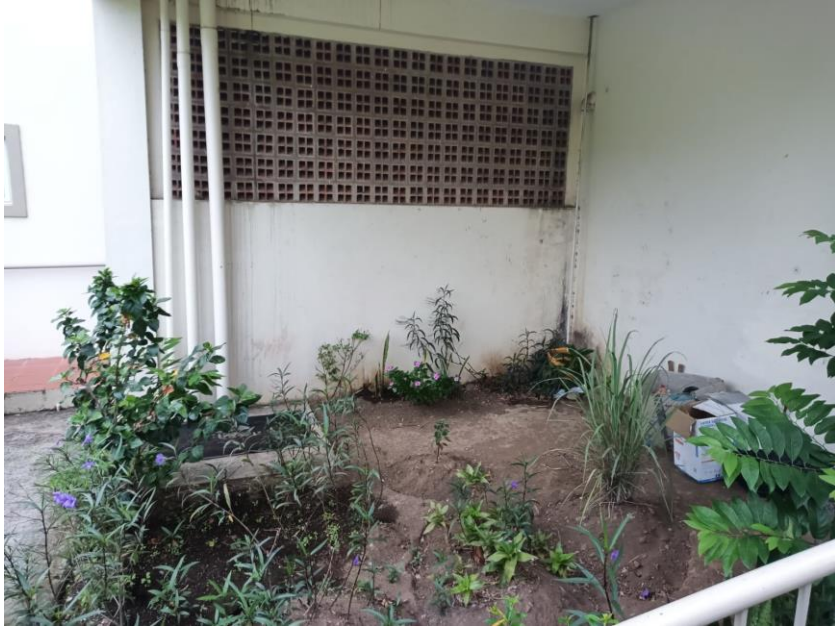
Figure 9. Wall to be demolished and open space to be renovated
