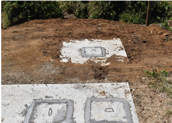
View of sealed septic /sewer system
