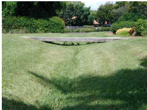
Figure 1 A Grassed Swale http://www.pbcgov.com/coextension/horticulture/neighborhoods/tips/images/swale.jpg
