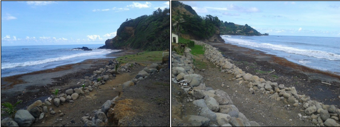
Figure 3.4: Creation of berms to reduce erosion
