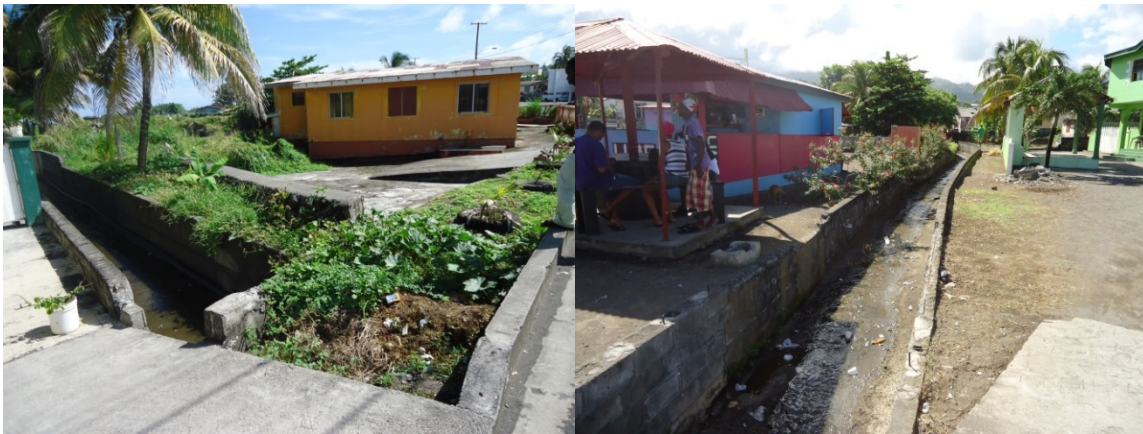
Figure 3.9: Rum Distillery waste stream looking seaward (left); looking inland (right)
