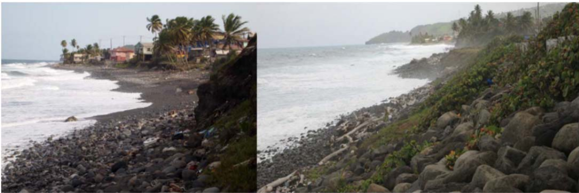
Figure 6.2: Irregular and undulating cliffs composed of cobble stones along Sector 1 (Source: Task 2 Report)
