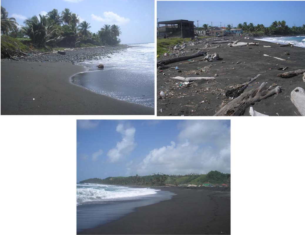
Figure 3.5: Beach Seaward of Georgetown playing field looking north (top); and looking south (bottom)
