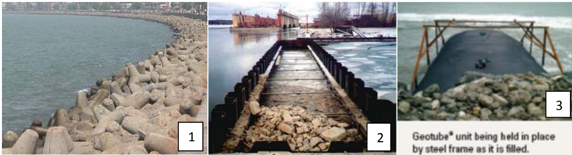
Figure 6.5: 1) Example of Interlocking XBlocs, 2) Example of Double-Wall Sheet Pile Cofferdam, 3) Example of Geotube
