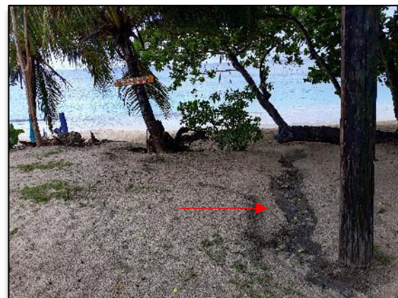
Figure 41. Red arrow points to an erosional stormwater gully from the roadside leading to the shoreline is a pre-existing issue.
