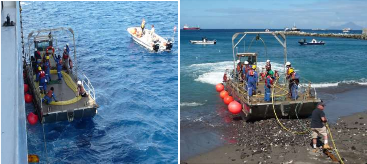
Figure 7. Cable transfer from cable ship to barge
