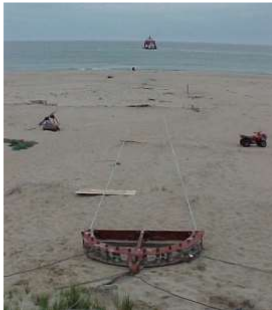
Figure 8. Cable pull from cable ship through beach quadrant
