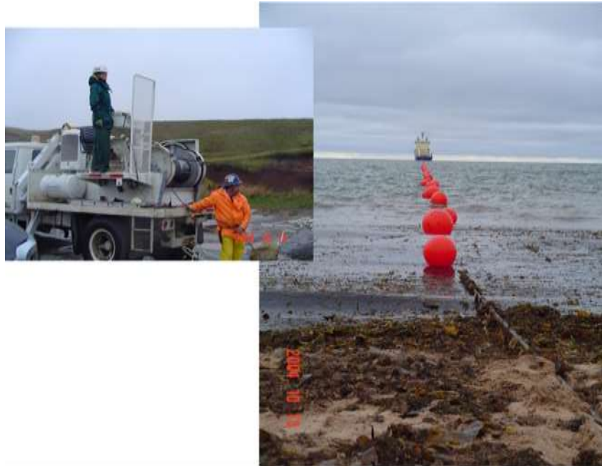
Figure 9. Floated cable pulled from the cable ship using a winch on the beach.
