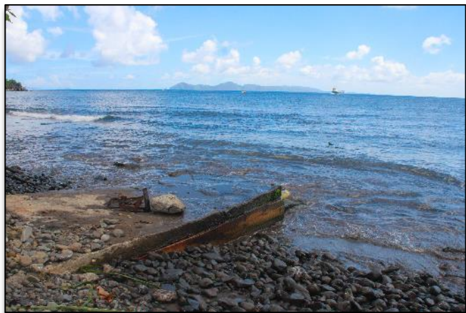
Figure 43. Existing beach manhole at Arnos Vale.
